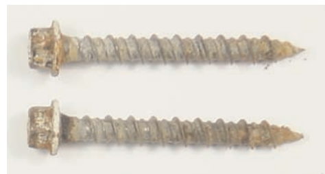
Untreated, southern yellow pine – some light rust and degradation
