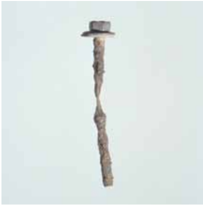
Coated carbon steel corrosion in a pitched roofing fastener
