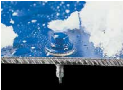
Washer must seal hole in weather skin
